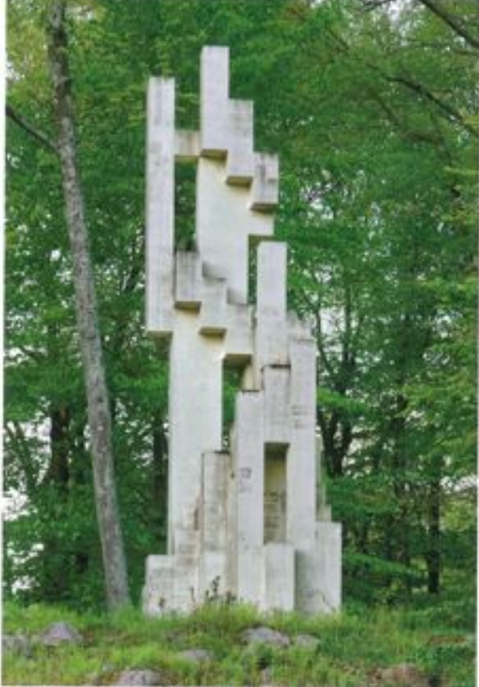
Repairing the 30-foot Lincoln Kirstein Tower is one of several conservation projects happening this summer at the Philip Johnson Glass House.
